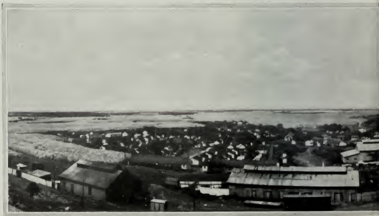
GENERAL VIEW OF PEARL
